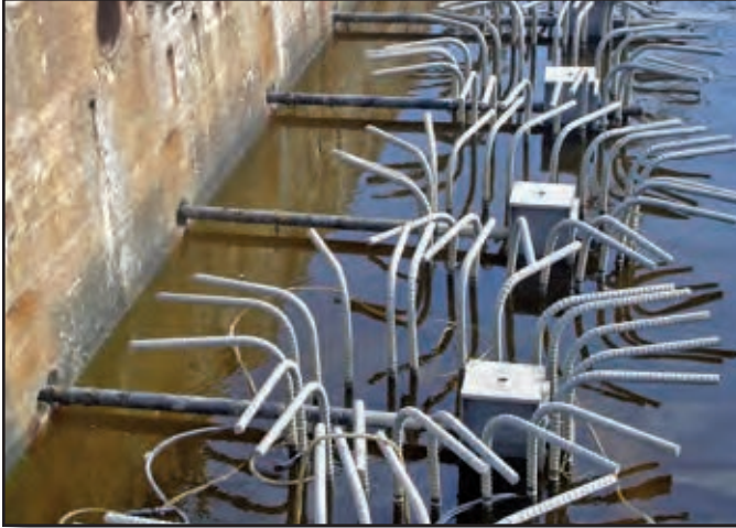
Project: Pier 3 Replacement Contractor: Weeks Marine Location: Portsmouth, VA
