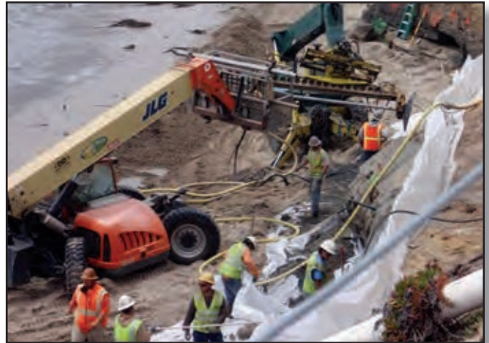
Project: East Cliff Drive Bluff Stabilization Contractor: Drill Tech Drilling & Shoring Location: Santa Cruz, CA
