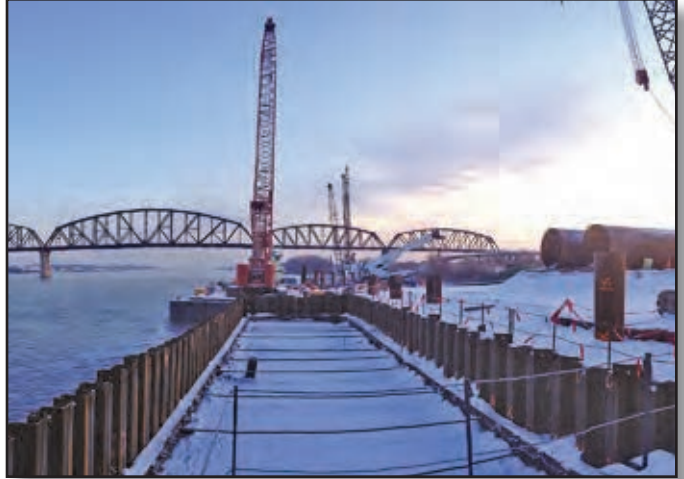
Project: Ohio River Bridge Contractor: Walsh Construction Location: Louisville, KY
